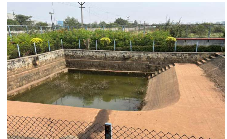
Rainwater harvesting pond
